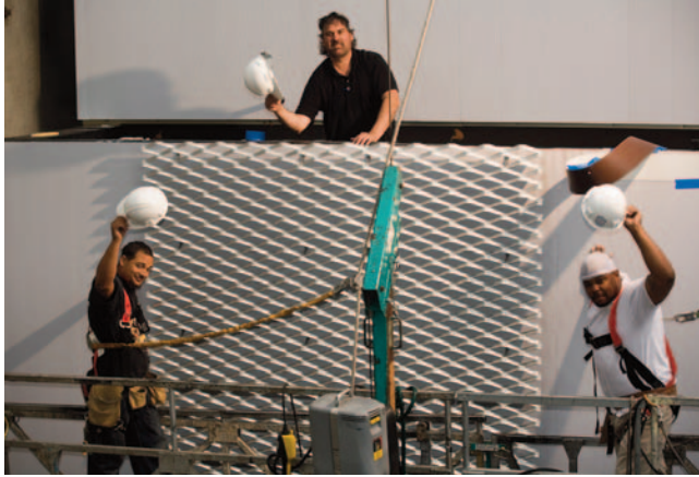
Workers begin installing building's mesh cladding
